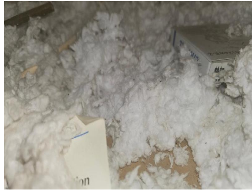
2190-3 Insulation Typical Interior
