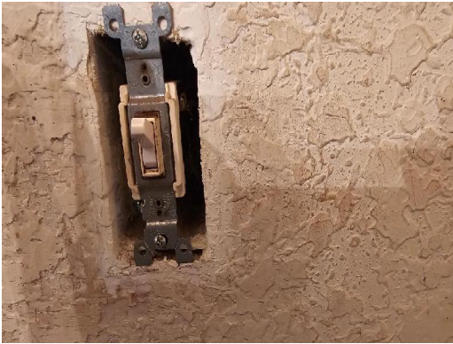
2190-2 Drywall/Joint Compound Typical Interior Walls/Ceilings
